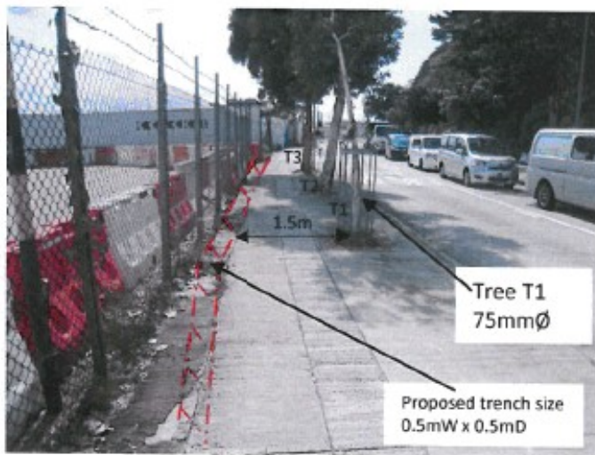
Photo 1: Horizontal clearance between trees and works area (with trees' diameter at breast height)
